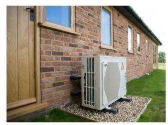
**Figure 91:** Air source heat pump unit located to the rear / side elevation of a dwelling, so to avoid its visual impact on the dwellings frontage and wider streetscape.
